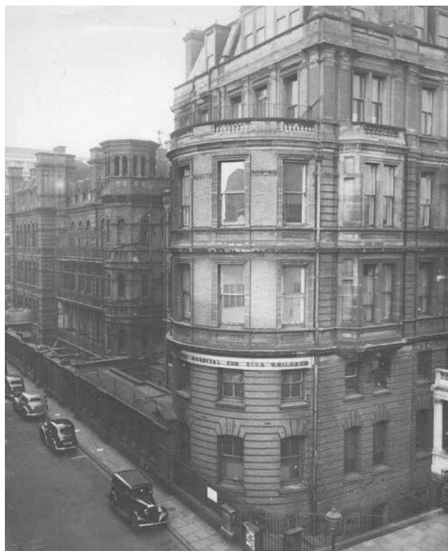
The 1893 South Wing (today's Paul O'Gorman Building) soon after the end of the Second World War.
